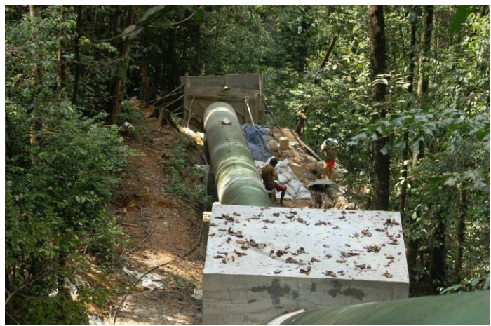
Pipelines at construction site inside Sripada Sanctuary
