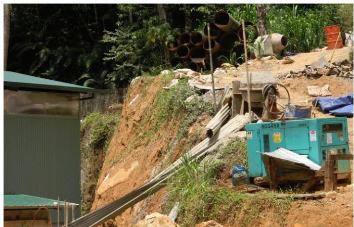
Construction site inside Sripada Sanctuary (Eli Hatha)
