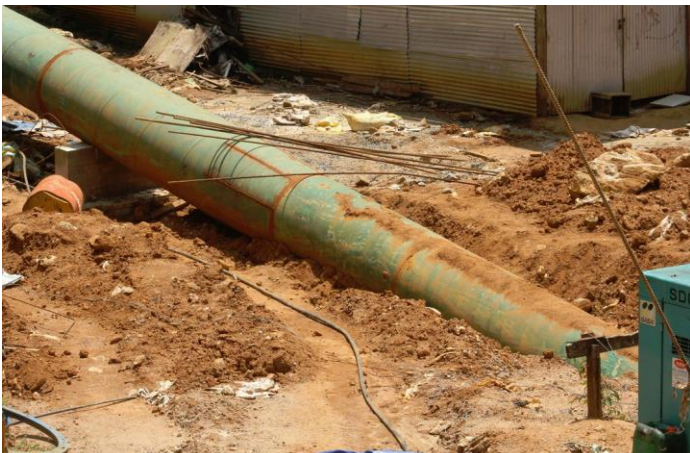
Construction site inside Sripada Sanctuary (Eli Hatha)
